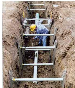
**Shielding** - Also called trench boxes or trench shields. These are structures that are placed in the excavation to prevent the sides of a trench from caving-in. The worker is only protected while in the "box." Some trench boxes can be moved as the work progresses. Heavy equipment must always be used to place the box or shield in the trench. The shield must extend at least 18 inches from the top of the slope of the trench.
